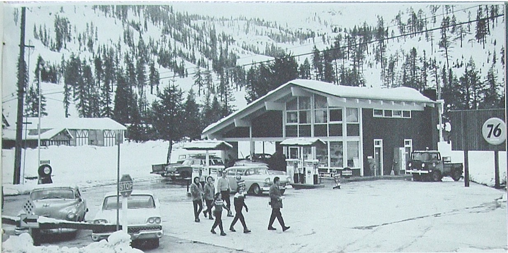
A dry oasis in the winter snows of Squaw Valley is our "76" pump island, radiant-heated fueling point for Olympic Games.
