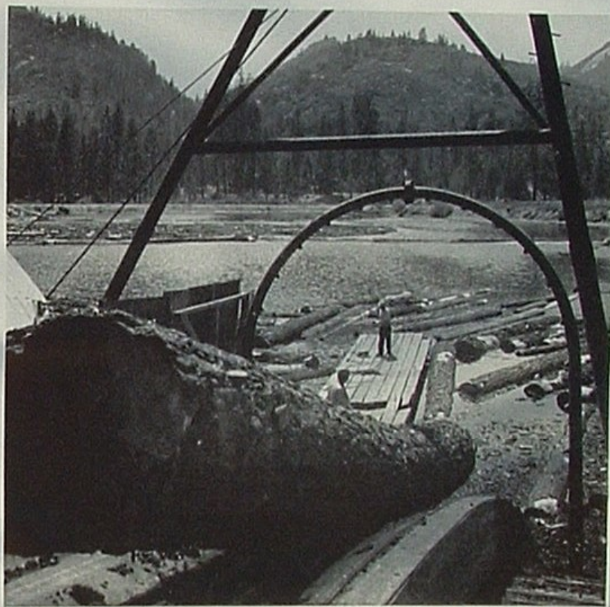
At right, sawmill operators select and guide logs to a chain conveyor, which lifts them into position for crosscut sawing into proper lengths.
