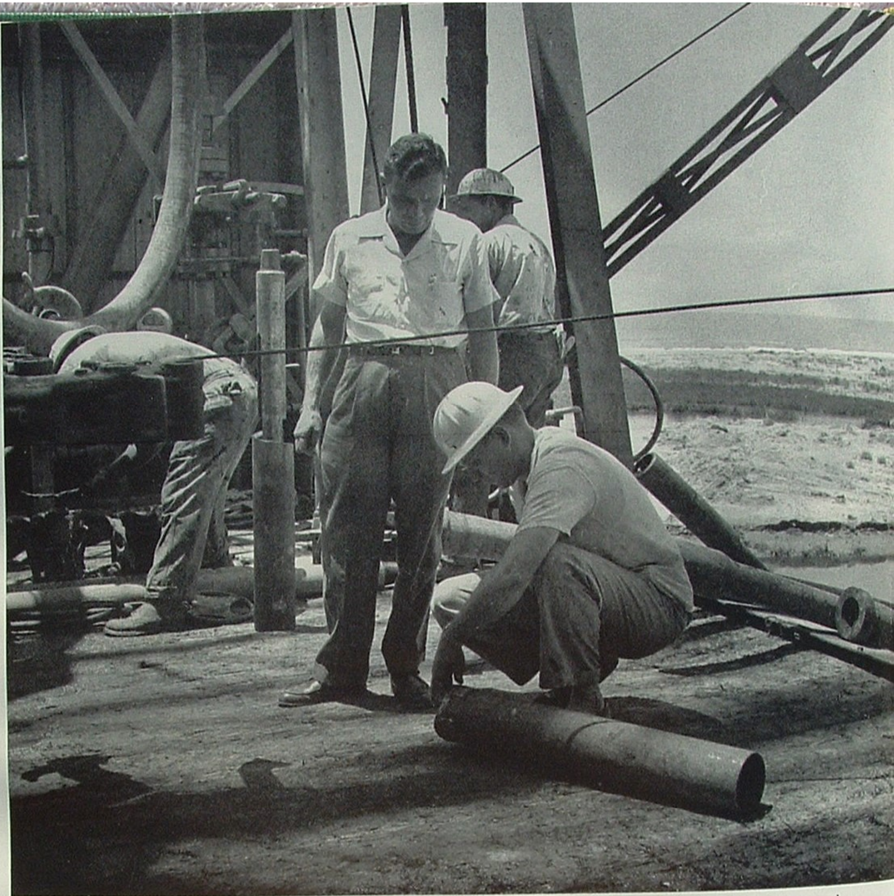
Even lucky drilling rigs have their troubles; down below the 17,000-foot mark the Bwana faced stuck drill pipe and a $100,000 fishing job. Foreman J. S. Buchanan and Engineer Joe Prosser examine part of the recovered "fish" worriedly.
