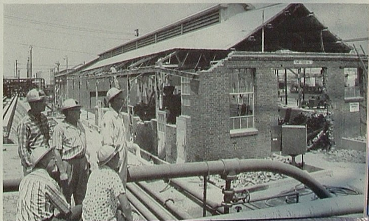
PUMP HOUSE NO. 1 at Los Angeles Refinery comes down after 40 years of service as the pumping "heart" of the big plant. It has been replaced by two new pumping plants, where dark and light oils are handled separately. At the "retirement party" were (standing, from left) H. O. Miller, Charles Robison, Alex Reckling; (seated) Web Francis and Robert Jones.
