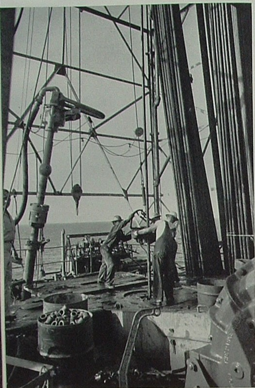
"Aboard B Platform the crew is installing tubing."
