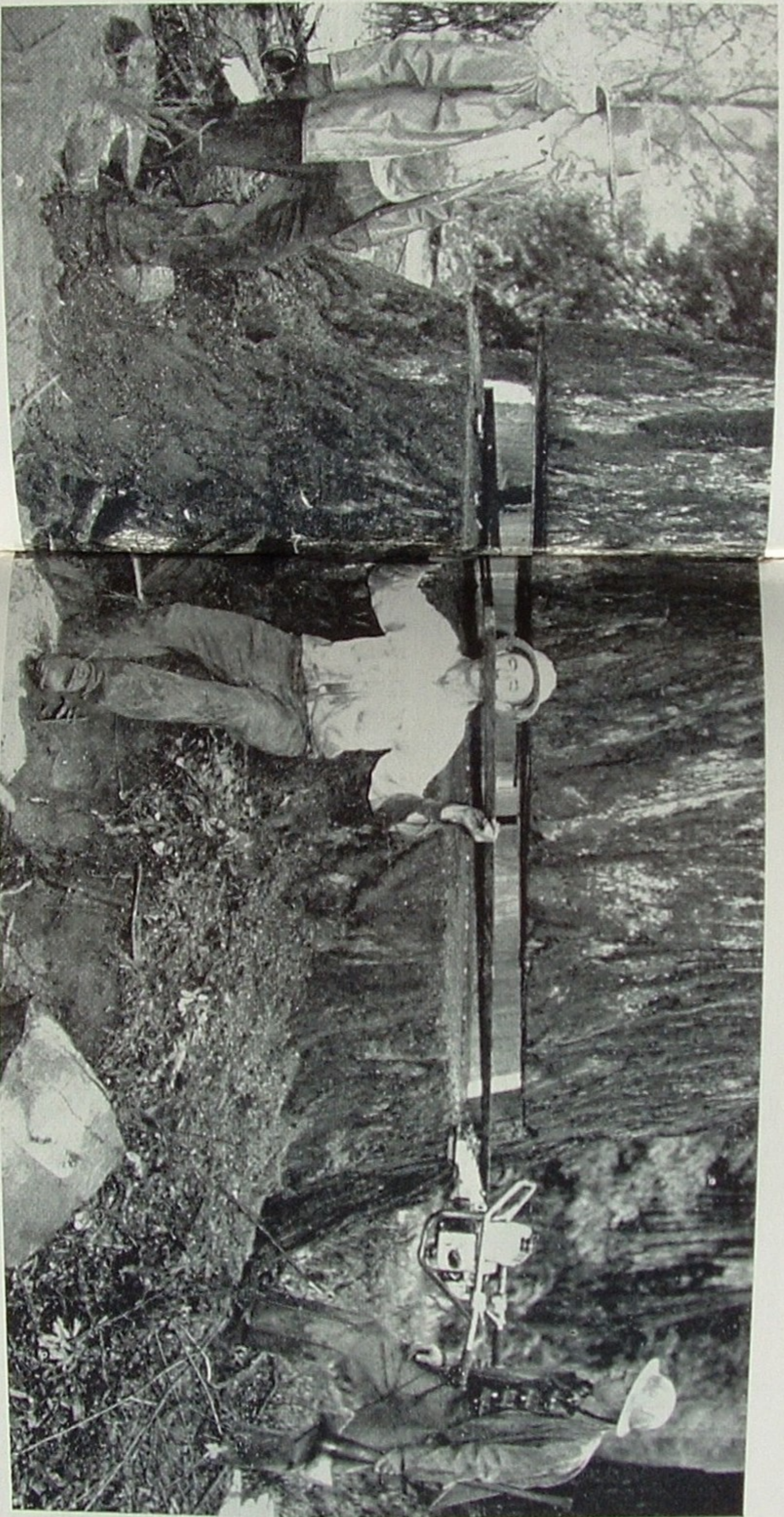
Great skill was required in making the undercut of this 11-foot diameter Redwood so that the tree would fall precisely on a pre-determined line, causing little damage to neighboring trees.
