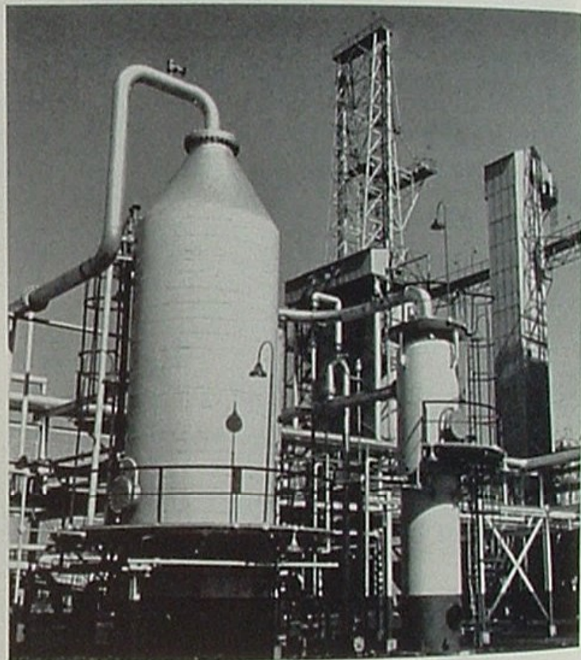
Our Santa Maria Refinery is a model of exceptionally clean coking. For example, the downward curving pipe (above), instead of venting pollutants to the atmosphere, carries them to a pair of sulfur plants (in photo at left). The latter do an excellent job of "scrubbing" the waste material and pay for part of their operation by recovering small quantities of elemental sulfur.
