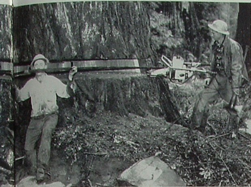
Great skill was required in making the undercut of this 11-foot diameter Redwood so that the tree would fall precisely on a pre-determined line, causing little damage to neighboring trees.
