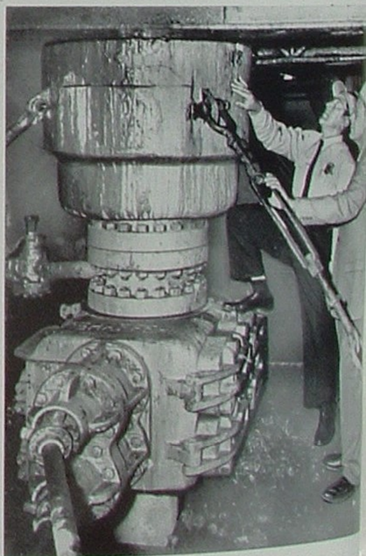
Fred B. Sevy, City Fire Bureau of Prevention inspector, checks the double safety of two blowout preventors. Upper is Hydril, which closes on round or square drilling pipe. Lower is a Shaffer, which will close on extremely high pressures. At right is James G. Schaeffer jr., superintendent.
