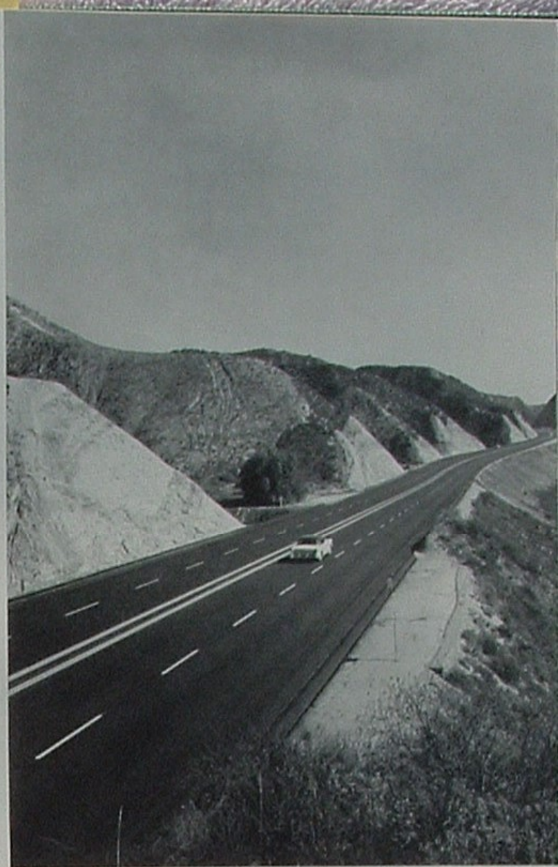
Knifing through some of the West's most rugged terrain, smooth asphalt roads are offering motorists better rides than were dreamed of in Arabian Nights.
