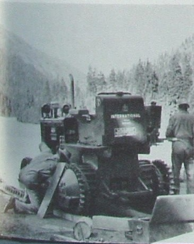
Contractor Henry Vanderwall of Idaho had to re-assemble his tractors following their airlift to job.
