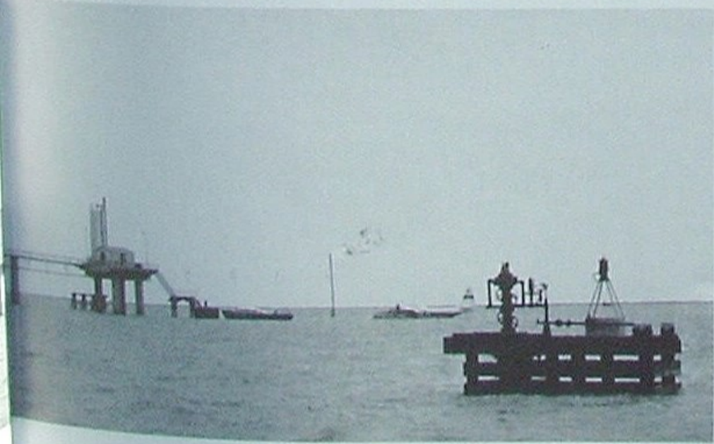
Our Caillou Island production platform on Timbalier Bay processes and ships oil from the new field where drilling record was made.
