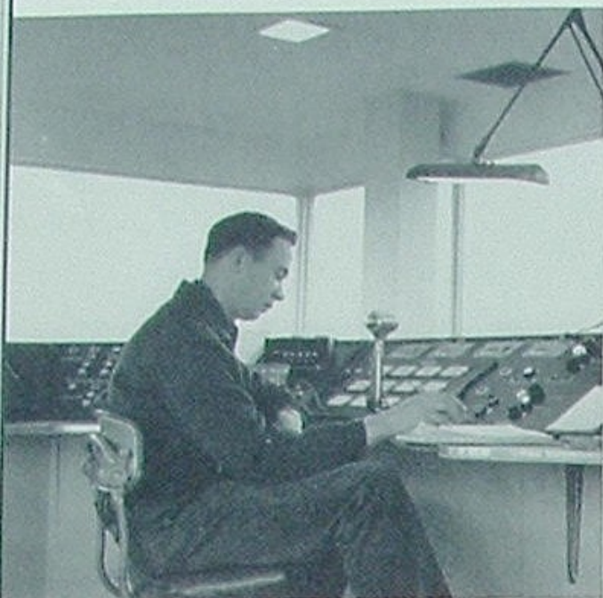
To Gauger Wayne Schaffer at Richmond, microwave brings finger-tip control of storage and line pumps.
