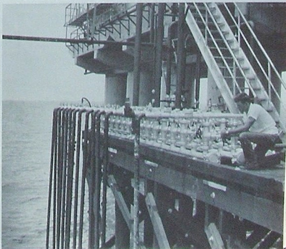
Each pipe rising from bay to manifold, explains Operator Curtis LeBeouf, comes from a producing well in the field.
