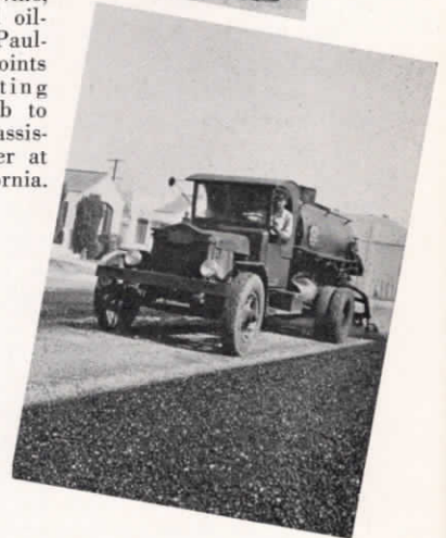
Above: Swampers must be nimble for their perch on the rear of the spreader truck is none too secure. Right: Having spread the heavy road oil on both shoulders of the road, the truck returns slowly, spreading a final coat upon the crown.
