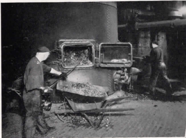
Above: The generator must be cleaned and recharged every ten hours. This is done from the plant's lower level. Right: During a gas-making period, which recurs at four minute intervals, the top of the super-heater is closed.
