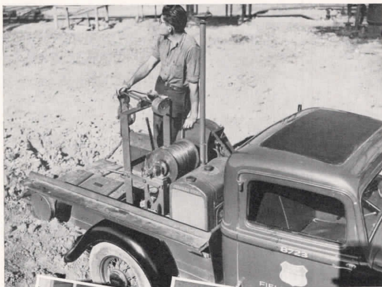
Left: This portable hoist is used to raise and lower the pressure bomb in the well. Basil Kantzer at the controls.
