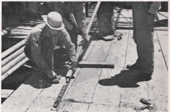
Below: Removing a core sample for inspection.
