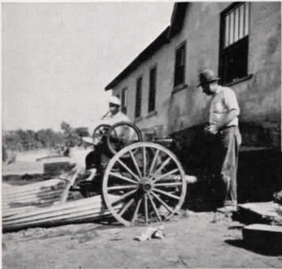
Below: Home off foundation in Atwood. Owner is pumping hundreds of gallons of flood water from cellar.
