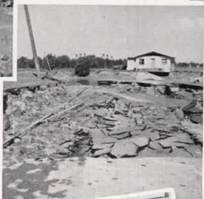
Below: Concrete meant nothing to the flood water. This photo shows a section of a street in Anaheim torn to bits. Note angle of house and telephone pole in background.
