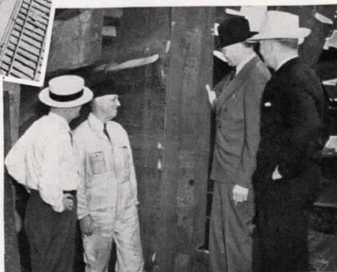
Below: Inspecting the welded wing bulkhead at forward end of the engine room. The wood shown in these pictures is merely staging and is, of course, removed when the steel structure has been completed.
