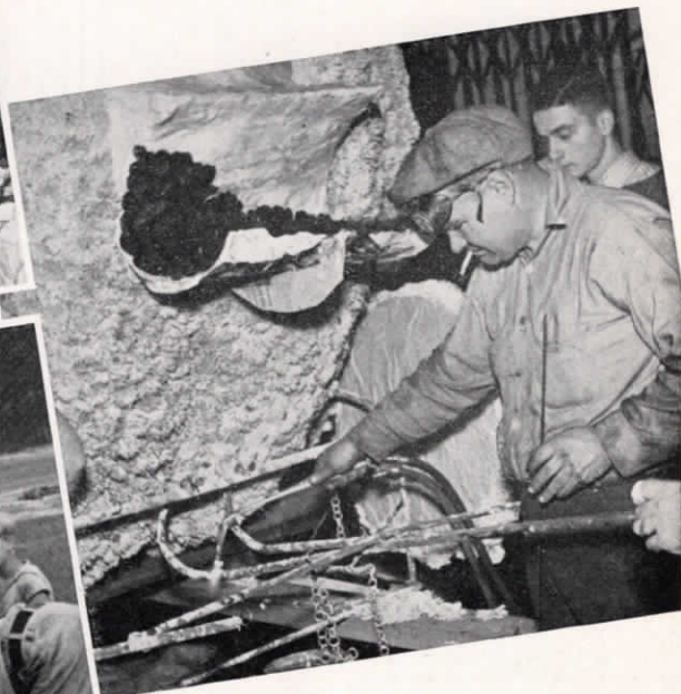
Below: Welding braces to strengthen the float.
