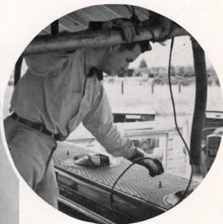
Right: Loading rack safety. Operator first attaches static wire to truck before loading it with gasoline.
