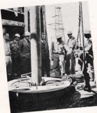
Committee conducts a safety investigation. Note members wearing safety helmets.
