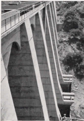
Above: Face of the Big Dalton Dam.
