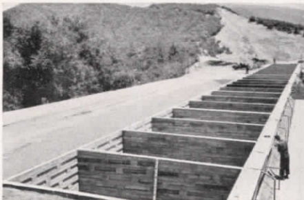
Right: Large lysimeters in the process of construction. Extreme right: A V-notched weir or flume used for measuring low stream flow.
