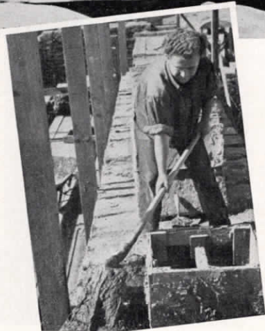
Left: The walls are reinforced with concrete columns, a form for one of which is shown here.
