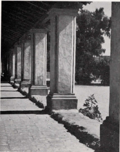
The straight columns at La Purisima Mission are distinctive, varying from the form used in other missions.
