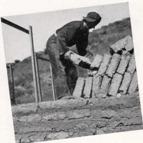
Left: The walls are reinforced with concrete columns, a form for one of which is shown here.
