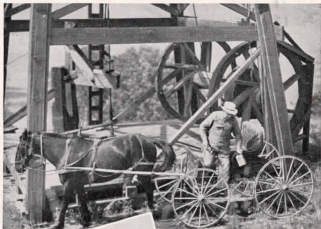
Left: A close-up of the lead line sampling operation; now almost as obsolete as the horse and buggy.
