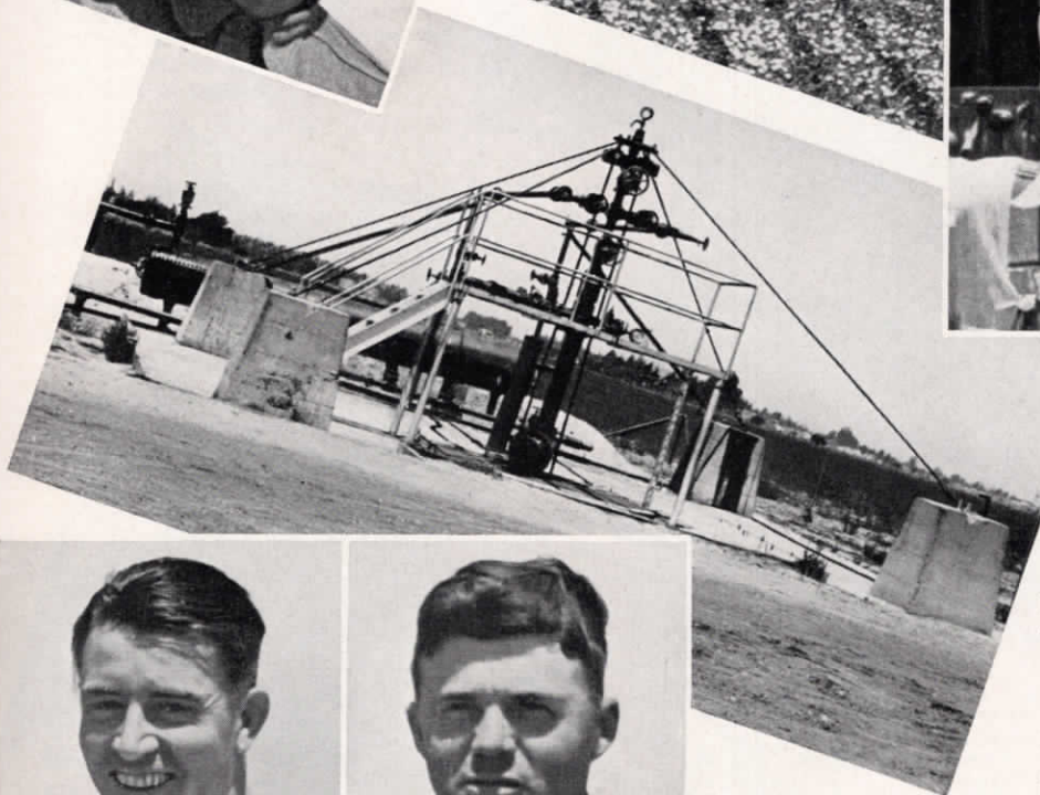
Left: Adam No. 1 well, the first big producer in the Santa Maria Valley Field, came in for about 2,500 barrels. Note that the derrick is gone, and nothing left but the "Christmas tree."
