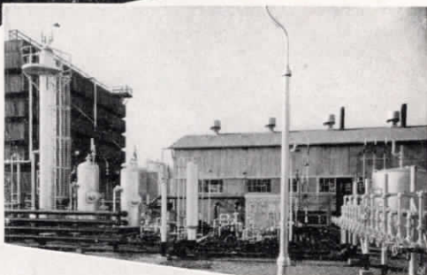
Right: Exterior view of the plant, showing stabilizer, cooling tower, and gas lift header.
