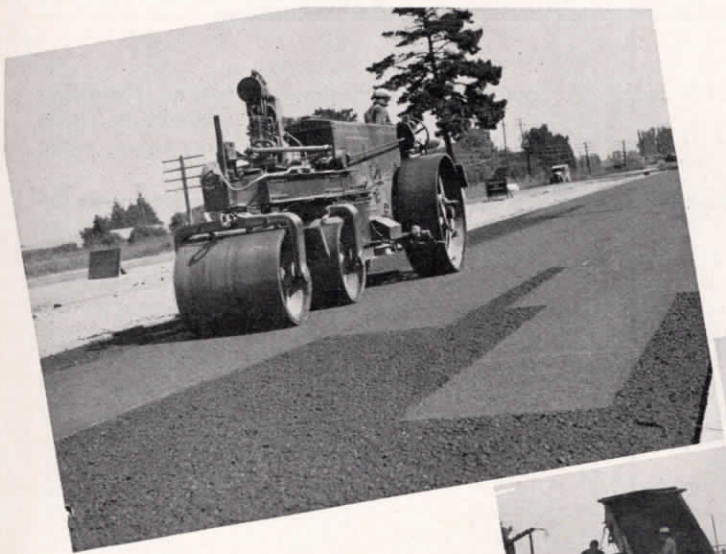
Above: Rolling the leveling course—the actual riding surface.
