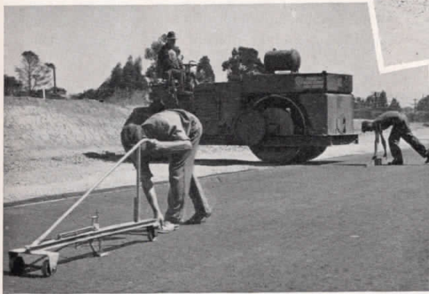
Left: Looking for high spots during rolling operations. The machine in left foreground detects irregularities in the surface.
