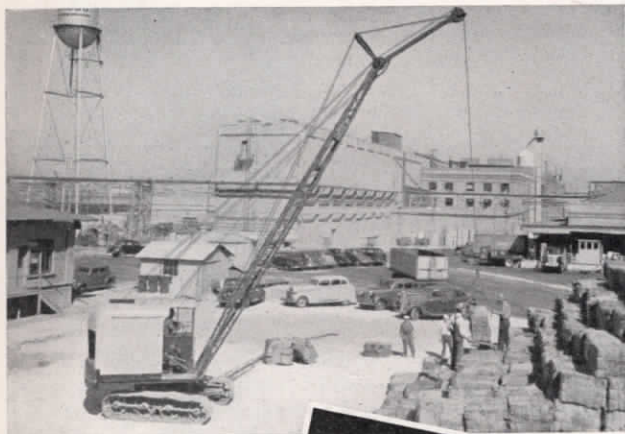
Left: Raw materials arrive at the PABCO plant, and are hoisted from dock to shore.
