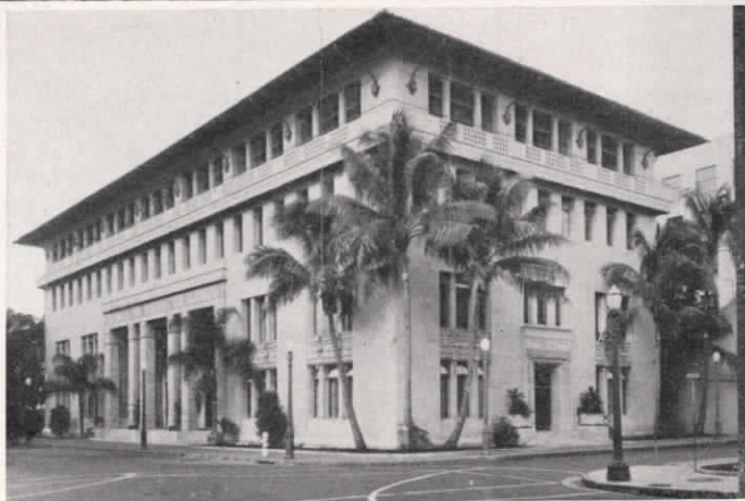
Right: in Honolulu, too, Pabco is a construction aid, as it is used both on the roof and in the basement of the Alexander and Baldwin building there.
