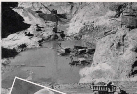
Above: The south cofferdam under construction.
