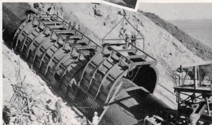
Below: A difficult section of siphon. Note that the inside forms are set under the reinforcing steel and an outside form is ready to be dropped into place. Then the forms are ready for concrete. Both inner and outer forms have been oiled.
