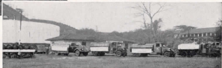
Above: The company's fleet of trucks lines up for a "Progress Parade."
