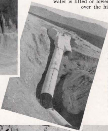
Below: A difficult section of siphon. Note that the inside forms are set under the reinforcing steel and an outside form is ready to be dropped into place. Then the forms are ready for concrete. Both inner and outer forms have been oiled.
