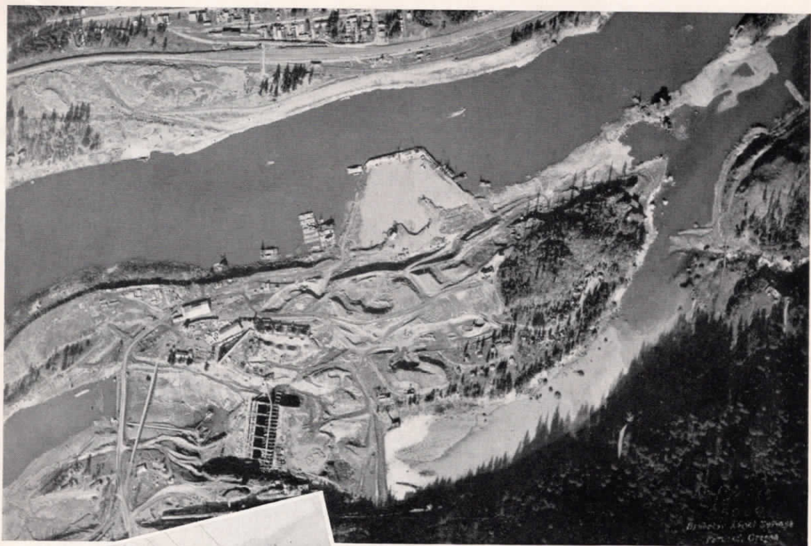
Above: Air view of Bonneville Dam project, showing, at right, partly finished power house foundation, and, at left, the coffer dam, where part of the main dam and spillway is being built.
