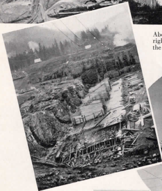
Above: Foundation of power house. Coffier dams have been built above and below the site to keep out the water during construction.
