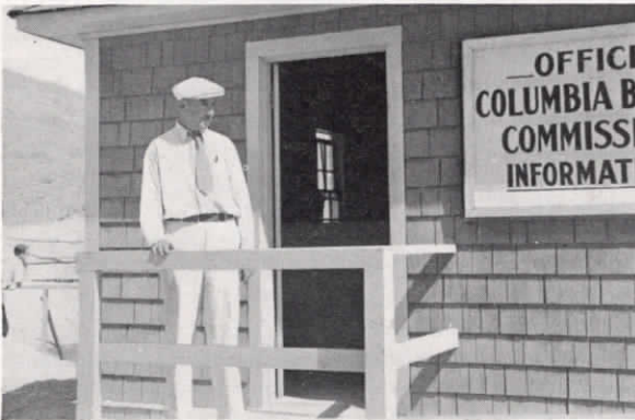
Above: R. J. Kugleman, former Union Oil Co. employee, now an engineer on Coulee Dam project. Right: The west concrete mixing tower and substructure, showing unusual length of supporting concrete columns.
