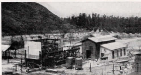
Torrey Absorption Plant.
