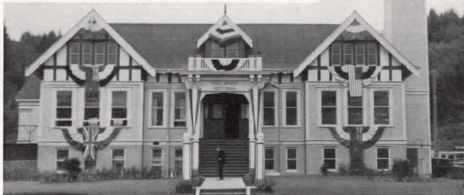
Port Moody City Hall.
