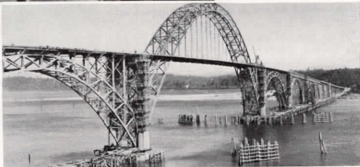
Right: The steel swing bridge across Yaquina River should be ready for traffic Oct. 1, 1936, and will mark the completion of the program.
