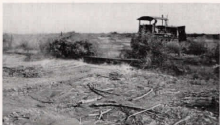
Clearing land with heavy rail.
