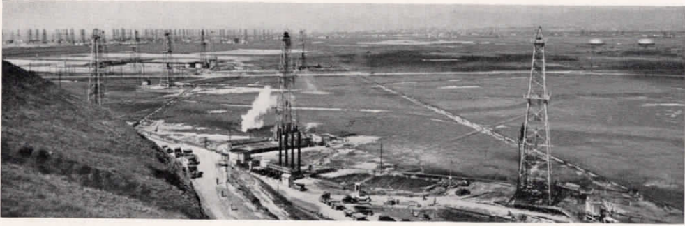
Union's Vidor wells Nos. 6, 8 and 7 in foreground in new Playa del Rey section.
