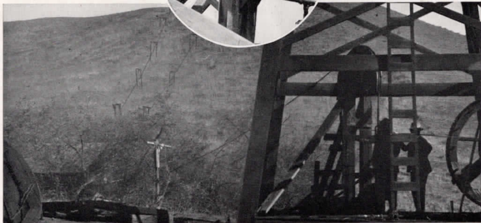
Dryden No. 1, exploration well at Bardsdale. Contrast this equipment with that of Grimes No. 4. Below: Old method of pumping at Bardsdale, with jack lines shown at left.
