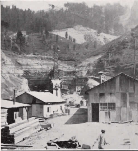
Compressors, tool sheds, and preliminary forms for ventilating equipment at west approach are shown at left. The diagram shows new tunnels, highway, and entrances from Bay cities. Below, grading west approach with ten Caterpillar "75's."
