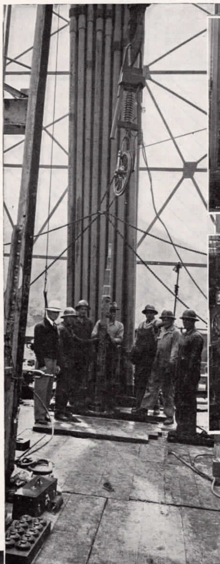
Left: Lowering the gun into the hole. Upper right: Back of special truck equipped for gun perforating, showing cable guide in center and several tiers of gun barrels on both sides. Lower right: Front of equipment of same truck, showing control board, loud speaking system and electric motors. Below: Result of test shot through 6 \frac{5}{8} -inch 26-pound, 8 \frac{5}{8} -inch 36-pound, and 10 \frac{3}{4} -inch 45-pound casing.
