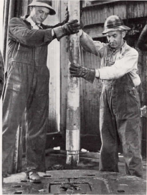
A core, taken with a regular formation coring device, is being removed from core barrel in the upper photograph, while at the right is core bit.
