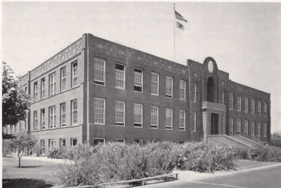
Administration building, company's Los Angeles refinery at Wilmington, Calif., which houses research department where Triton was born in the test tube and upon the roof of which the experimental plant, that first produced Triton, was built.
