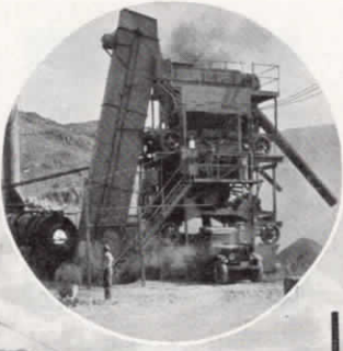
114-ton per day asphalt batch mixing plant operated by Basich Brothers is shown at left, and below, 220 horsepower Diesel generator which supplies power to operate mix plant.
