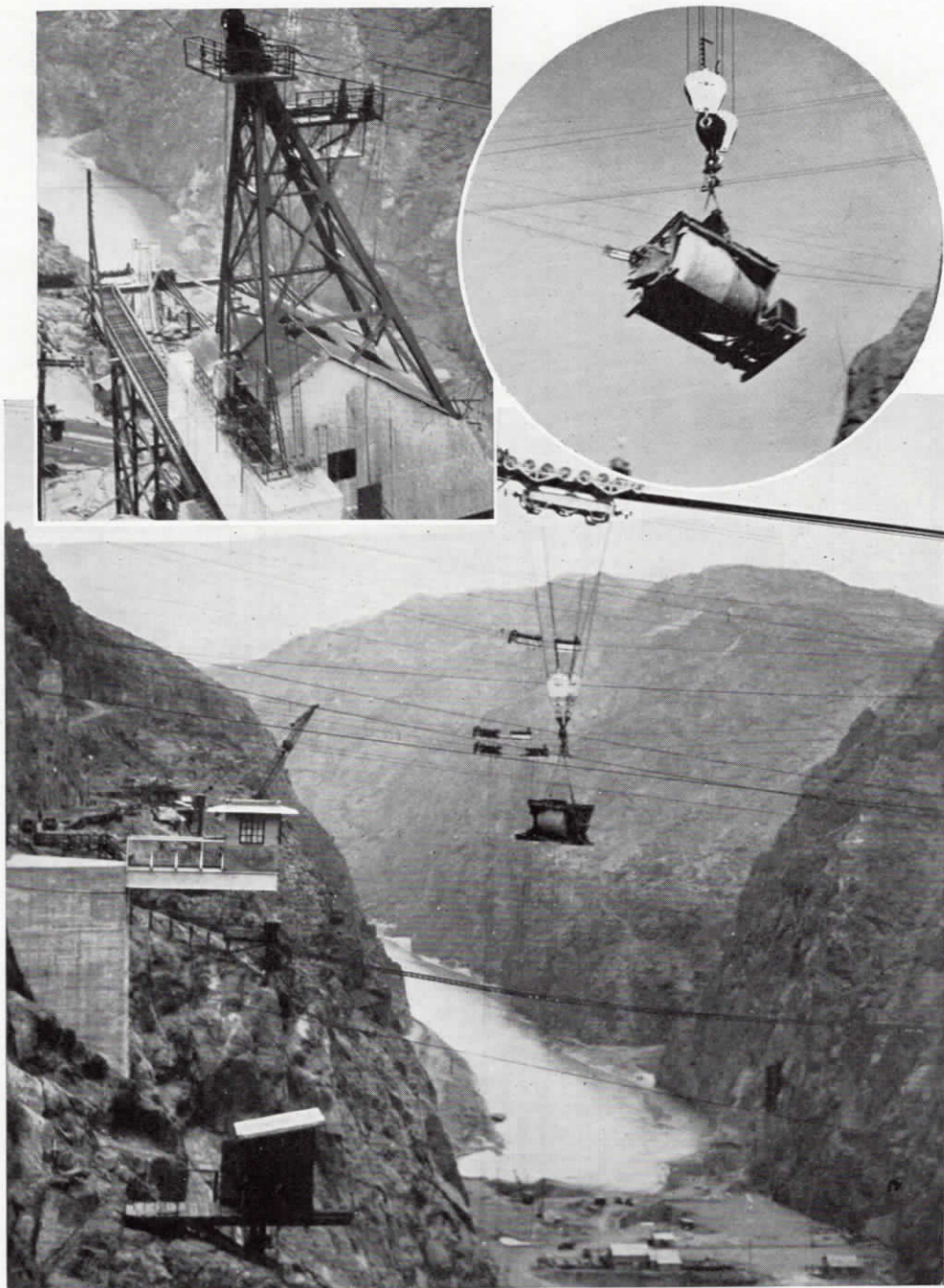
Cableways are playing the largest single part in the present work at Boulder Dam. Top, left, inset, one of the mobile, counter-weighted cableway anchors with control house, from which trolley and lifting slings are manipulated. These anchors may be moved, by their own power, along a track for distance of nearly 400 feet in order to accurately spot a concrete conveyor over the proper dumping location. Circled inset, one of the 8-cubic yard conveyors being lowered in the canyon. The large government 150-ton cableway, operated from control house jutting over canyon wall at the left, is shown above. Note the 6-cable suspension and multi-wheeled trolley. Trolleys of three of the five other cableways which span Black Canyon over the damsite, may be seen in the background. This view is looking upstream from observation point.
