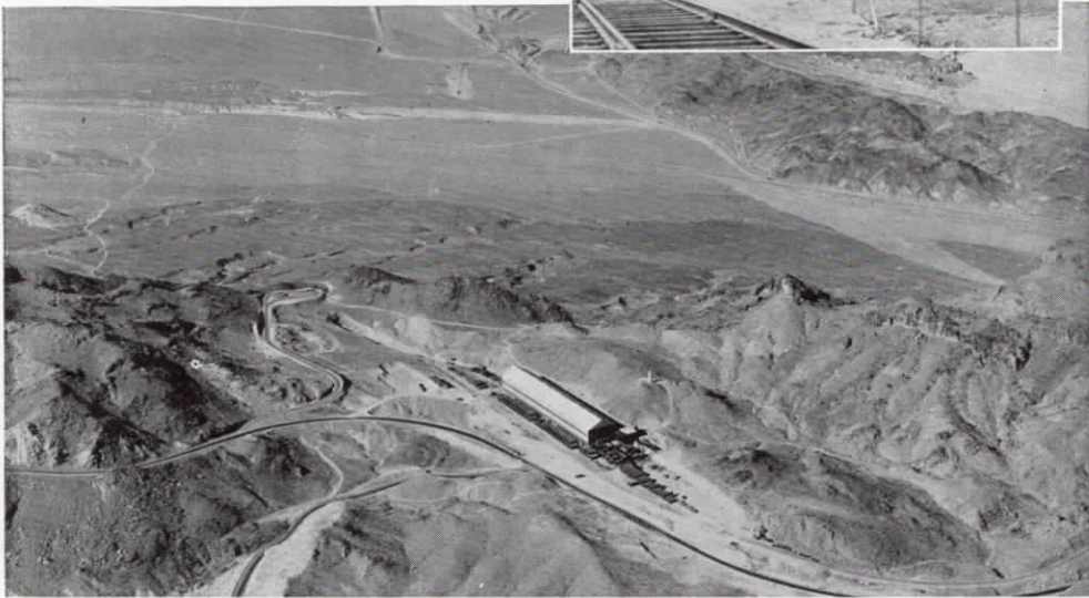
Stored sections of 30-foot diameter pipe, to be used in lining penstock tunnels, are shown in top photograph. In the lower picture is fabrication plant of Wilcox and Babcock, where all steel pipe for lining tunnels is cold-rolled in sections. Rail lines and highway disappearing in lower right of the picture lead to top of the canyon wall overlooking the damsite.
