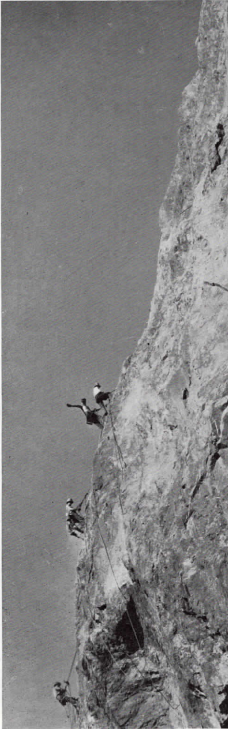
"High Scalers" chipping loose rock from canyon wall.
