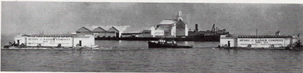
Henry J. Kaiser Company concrete mixing barges being towed to Eastbay crossing piers
