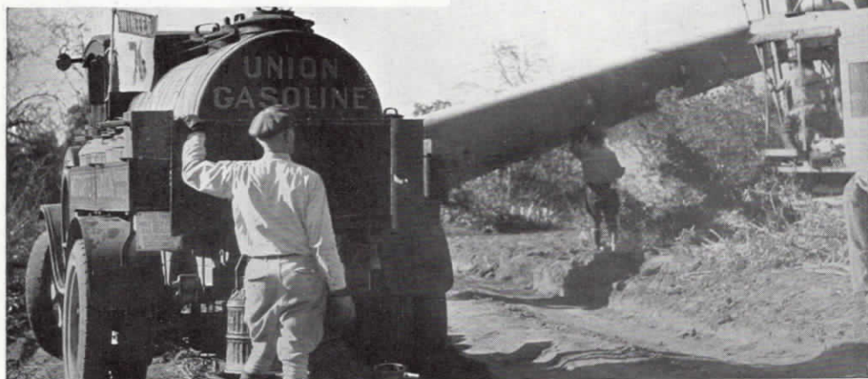
Laying 36-in. pipe line from Pine Canyon dam.
