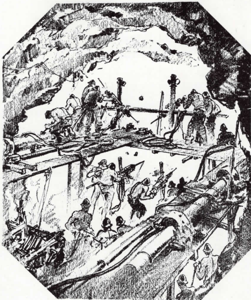
Boring through 13 miles of granite in the San Jacinto tunnel as dramatically sketched by Charles H. Owens and reproduced through the courtesy of Los Angeles Times.
