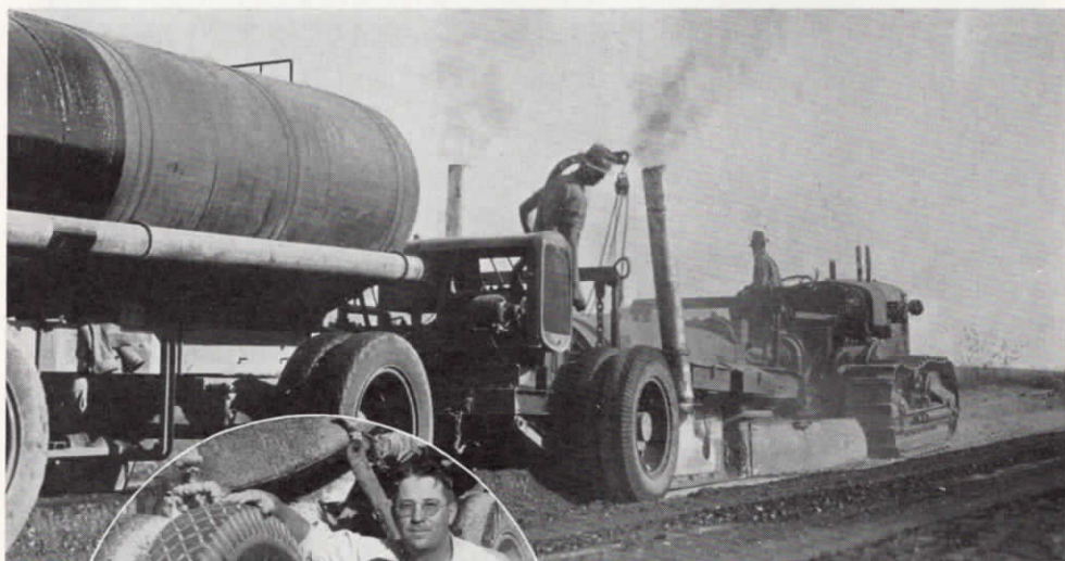
Roadbuilding equipment of Clyde W. Wood Company at work on highway paralleling the aqueduct. In a continuous operation this machinery picks up dry road material, passes it through a furnace in which it is mixed under extreme heat and pressure with hot road oil, and then dumped back on road. Scraper and grader level off the composition, and traffic pounds it into a highly satisfactory roadway. Clyde Wood is shown in inset at the left.
