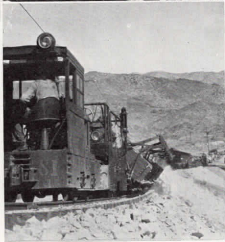
Portal of Hayfield Tunnel No. 2, with new type mucker shown at work. It scoops up material jarred loose in dynamiting and conveys it on an endless belt into dump cars. Picture at the right shows muck cars dumping rock removed from driving face of Cottonwood Tunnel.
