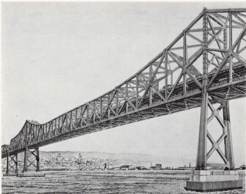
One of the cantilever spans of the Eastbay crossing, as completed by the artist, showing Oakland in the background.
