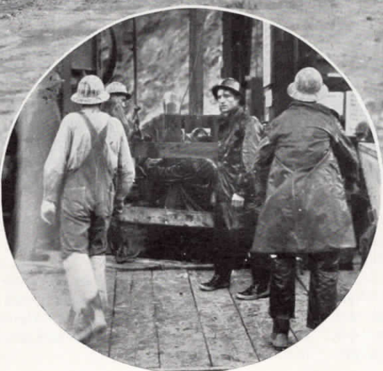
Workmen are lowering 22-inch air-vent tubing into shaft of Valverde tunnel in top picture. Potrero shaft heading of the San Jacinto tunnel is indicated in the large photograph. This shaft drops vertically more than 850 feet to reach tunnel level. Shaft workers may be seen in the circle at the left coming out of Potrero shaft in skip bucket as the shift changes.
