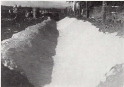
A new experiment is being made by the Hawaiian Sugar Planters' Experiment Association in the use of a mixture of emulsified asphalt and baggass (the residue left from cane stocks) with certain other ingredients, known only to the Experiment Association, in lining irrigation ditches. The mixture is applied with a spray with the results shown in the above photograph.
