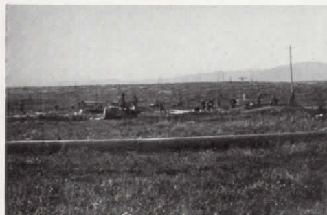
Injecting warm water in the ground to thaw it for dredging.
