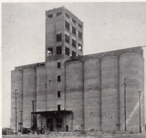
Farmers National Warehouse Company's latest grain elevator recently completed at Spokane, Washington.
