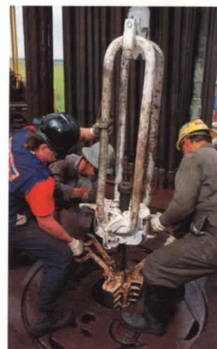
Clockwise from top left: a gas contact tower removes water from unprocessed natural gas at Unocal's Lake Pagie production facility; heater treaters at the West Starks production plant warm natural gas to separate various hydrocarbon components; field workers "make hole" at the onshore North Freshwater Bayou field.
