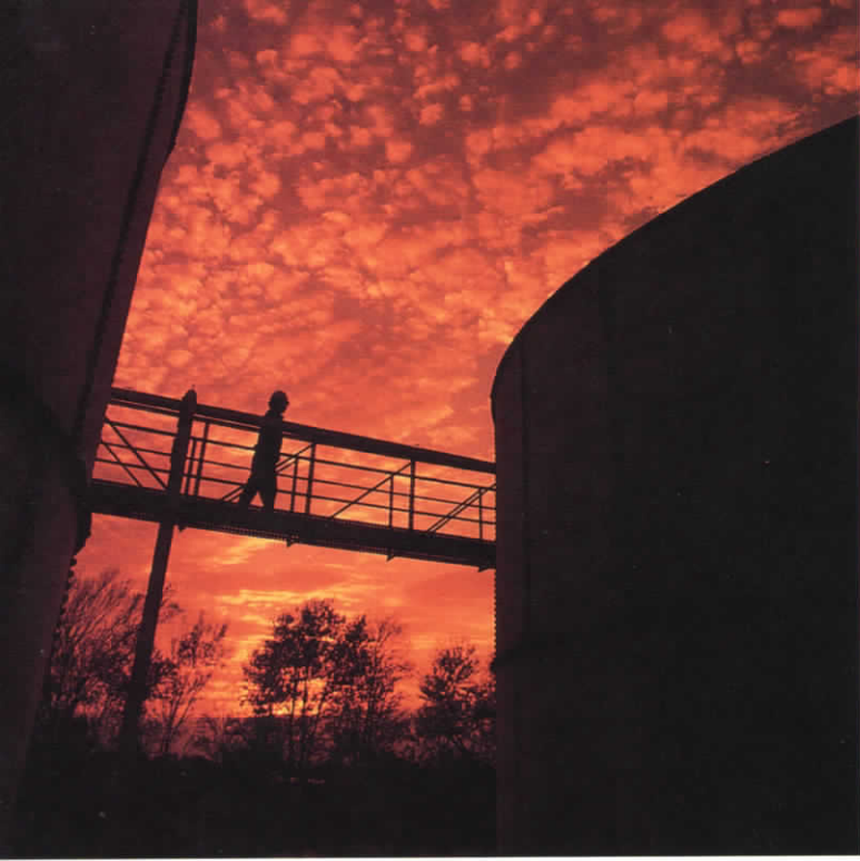
Above, a worker inspects oil storage tanks located in Unocal's Lake Pagie field in Southern Louisiana. The company made eight new hydrocarbon discoveries in the Gulf Coast area in 1990 and completed several development projects that added more than 100 million cubic feet per day of gas production.
