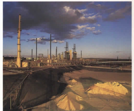
Clockwise from above: the Unisulf plant at the company’s Santa Maria refinery removes sulfur from refinery gases; exploration drilling offshore Thailand; steam injection in Unocal’s Cymric field, central California. Environmental systems, exploration technology and enhanced oil recovery are three focus areas of the company’s research effort.
