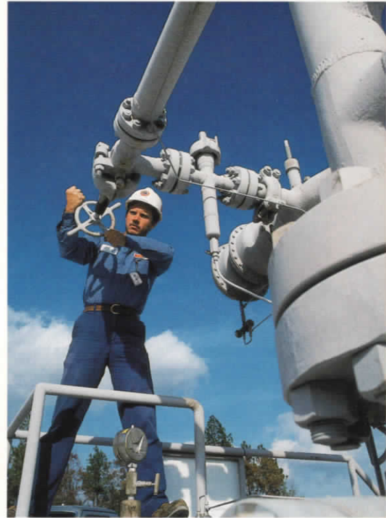
The Chunchula field produces about 9,000 barrels of condensate and 50 million cubic feet of natural gas per day. Production goes directly from the wells to the Chunchula gas processing plant, a portion of which is pictured at left. Top, a row of product storage tanks at the facility. Above, an employee adjusts a wellhead valve to regulate flow.
