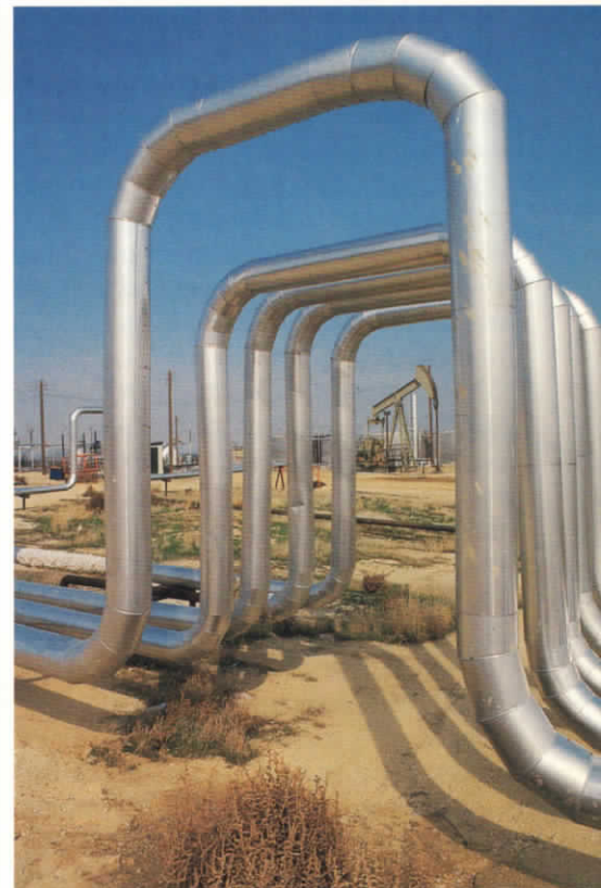
Located in California's San Joaquin Valley, Unocal's Cymric field was the site of the company's first attempt at steam injection. The method is now a widely used enhanced oil recovery technique.
