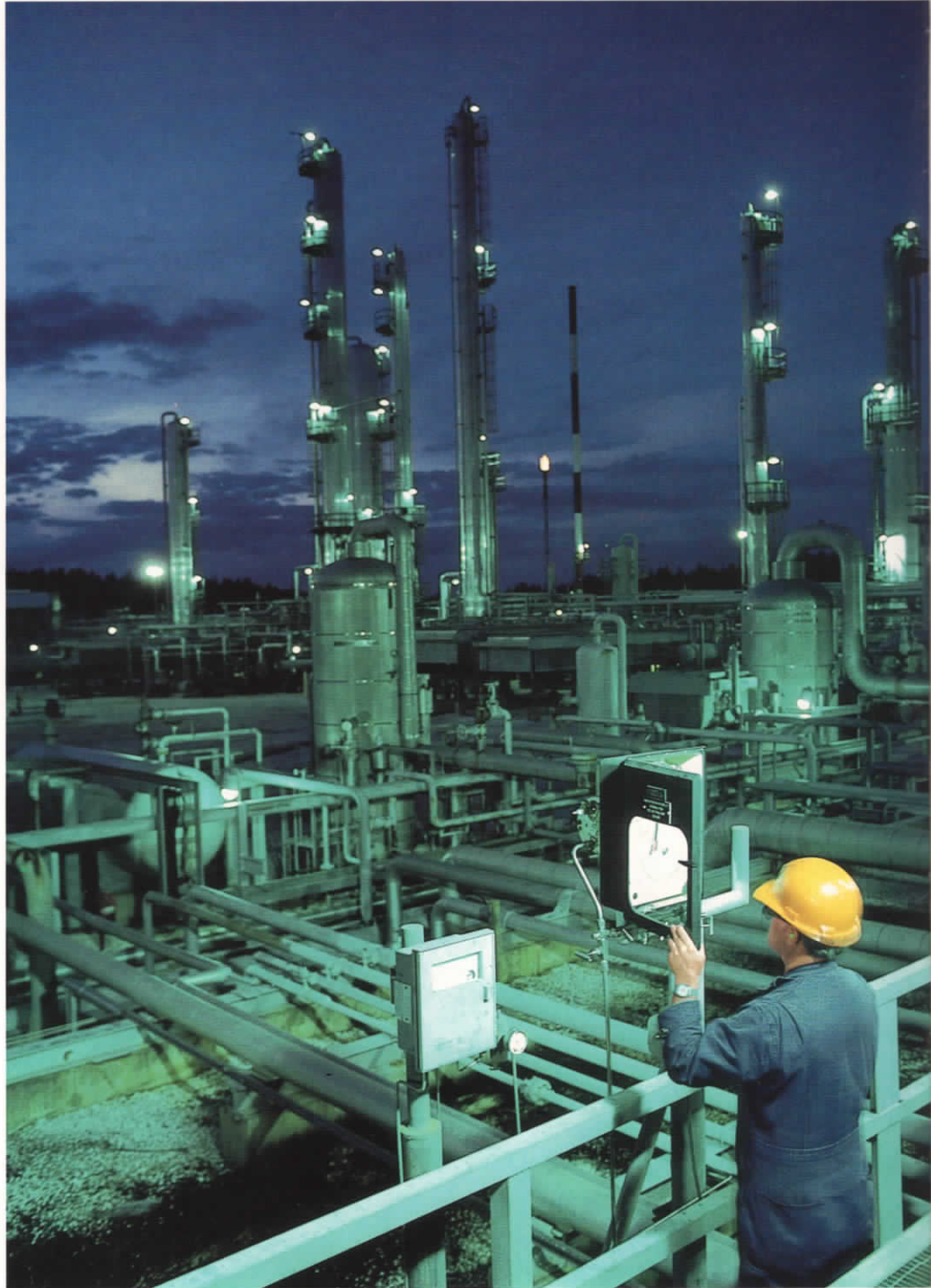
Right, a worker changes a chart in one of the processing plant's pressure recorders. Top, a drilling rig at work in the Chunchula field, discovered by Unocal in 1973.
