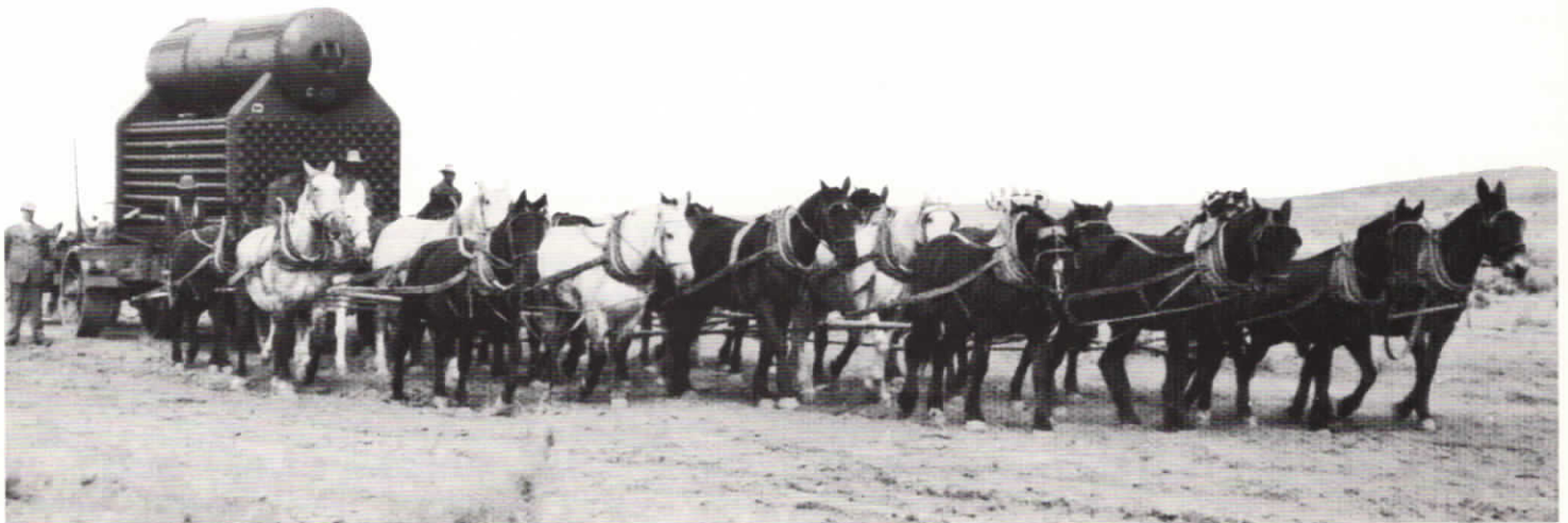
Below, a mule team transports one of the steam boilers to a pump station site in 1909. Opposite, one of the pipeline’s construction crews poses.
