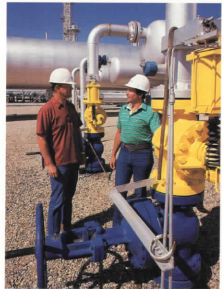
Clockwise from above: Project manager Dave Peters (right) and plant and field foreman Jay Axtell tour the plant grounds; one of the Lisbon field's wells; Peters and Axtell pause above a pair of liquid propane storage tanks.
