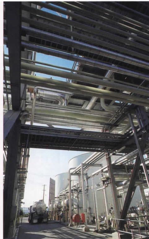
The cogeneration plants enable both refineries to produce their own electricity and steam. They also can keep the refineries operating in the event of a power outage. Pictured here is the San Francisco refinery's cogeneration plant.
