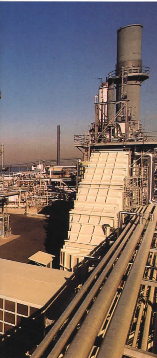
The cogeneration plants enable both refineries to produce their own electricity and steam. They also can keep the refineries operating in the event of a power outage. Pictured here is the San Francisco refinery's cogeneration plant.
