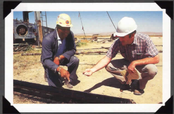
Inspecting the results of a reformation.
