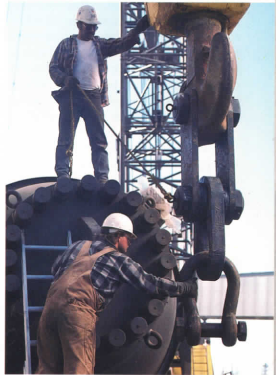
Clockwise from top: Workers inspect a dismantled "granulator tire," used in the urea production process; securing one of the new urea process vessels to a crane; a section of the Kenai plant, looking south.
