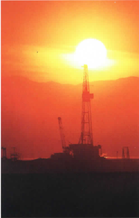
A drilling rig "makes hole" at the company's Salton Sea geothermal project. Scaling and corrosion problems caused by the area's highly saline geothermal fluids have been overcome through an intensive research program.
