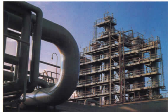
Clockwise from left: Alkylation unit at the Beaumont refinery; the Chicago refinery's Unisar, which removes aromatics from jet fuels and solvents; Beaumont's lube oil extraction unit.
