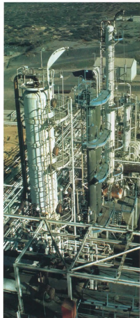
Distillation tower, Santa Maria refinery.
