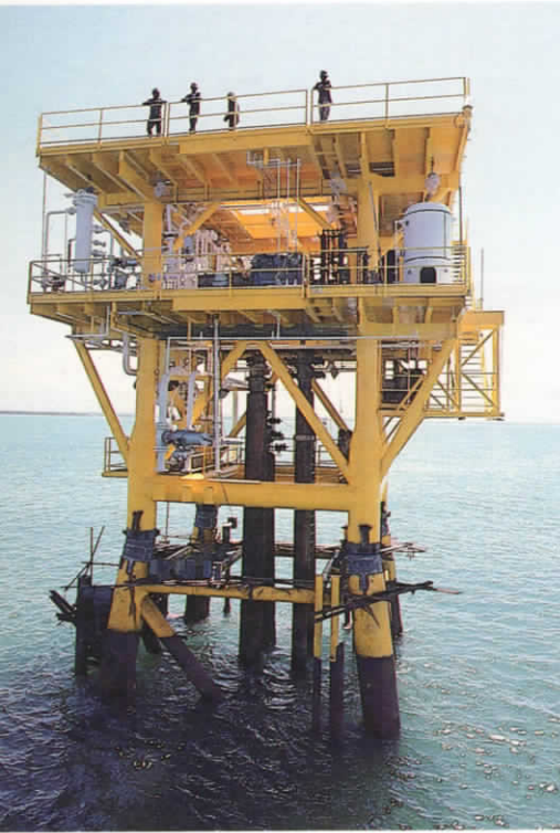
By early 1986, total production from the Yakin complex is expected to reach 15,000 barrels per day.
