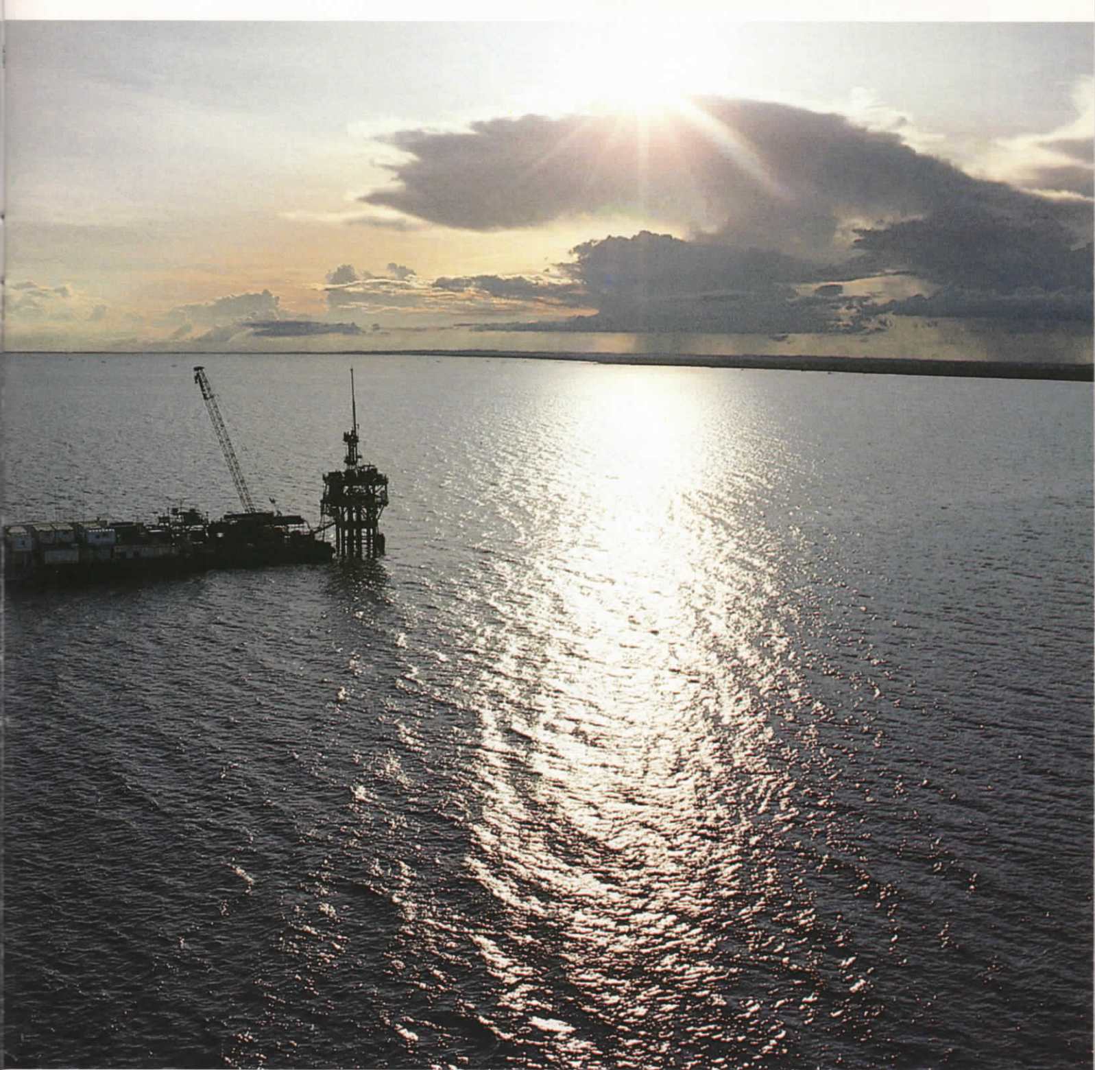
Drilling underway in the Yakin complex, offshore East Kalimantan. Unocal's Indonesian operations now span 15 successful years.
