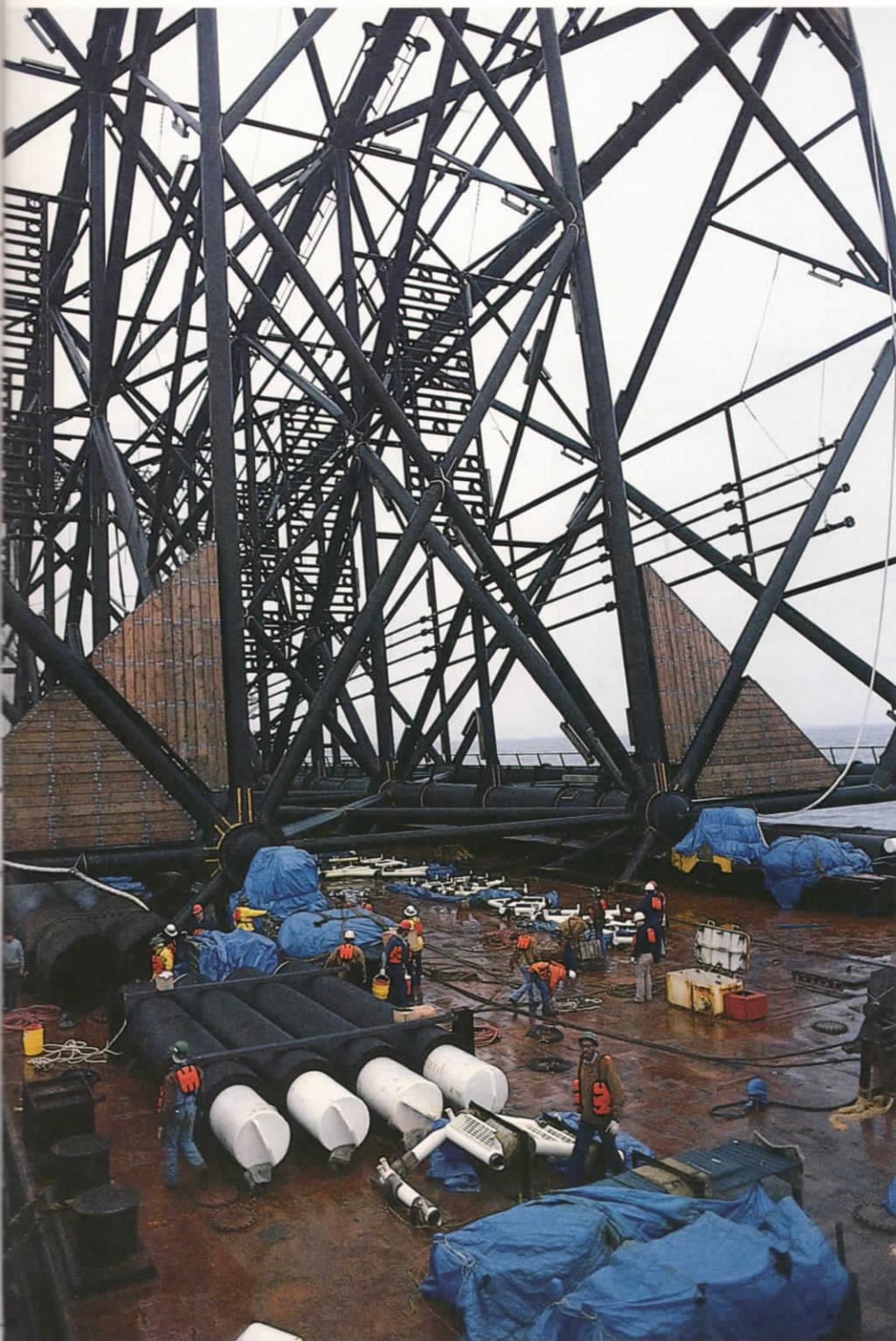
At left, Rich Keller (with camera) discusses strategy with a member of the Sarita crew during the setting of the platform jacket. The decks were installed about two weeks later.
