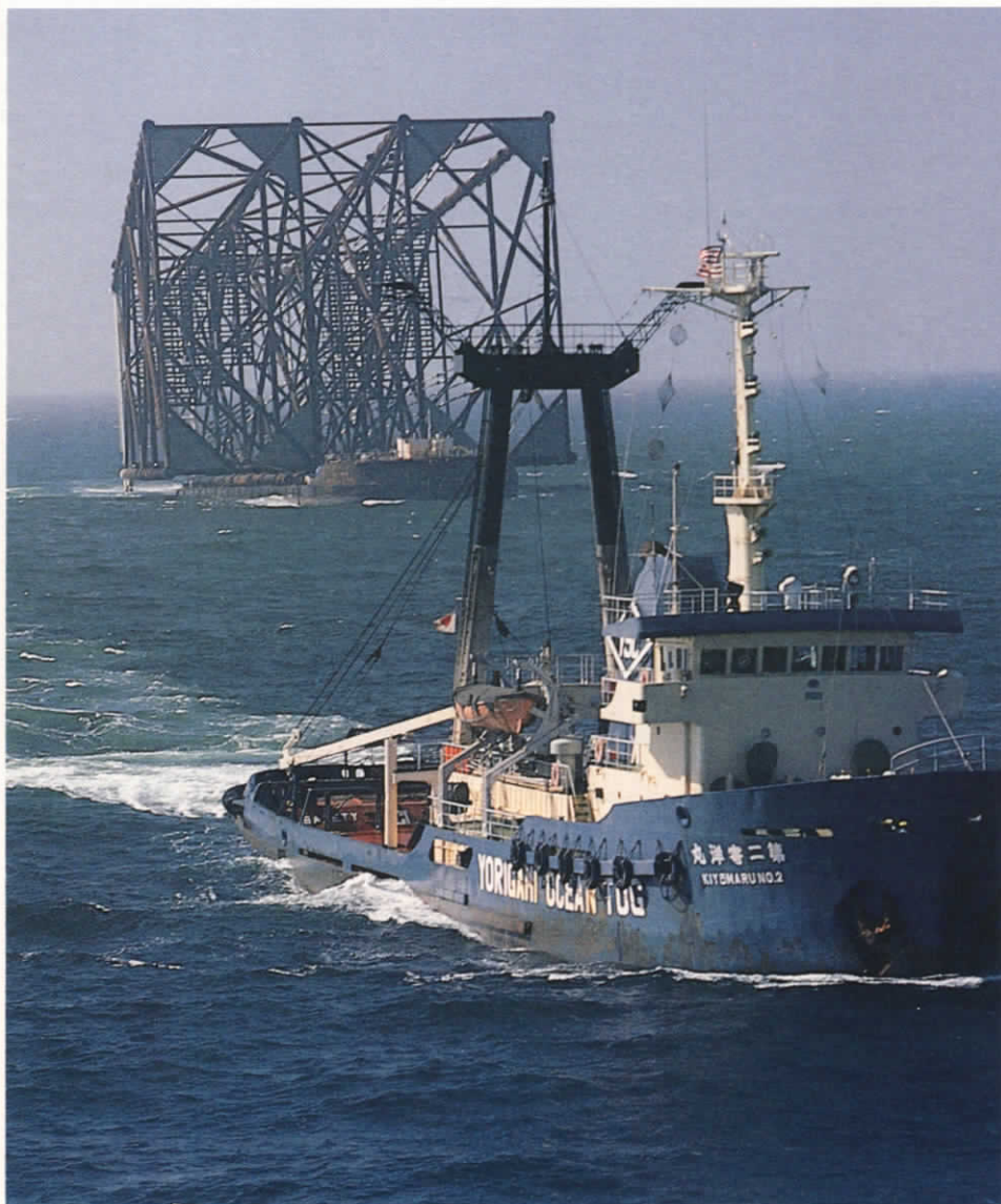
Arrival: Platform Irene’s jacket dwarfs the barge that tows it to its launch point offshore California. At top, the jacket is angled towards the sea in the first stage of the launch. Once secured to the ocean floor, the jacket is ready to receive its decks (above).
