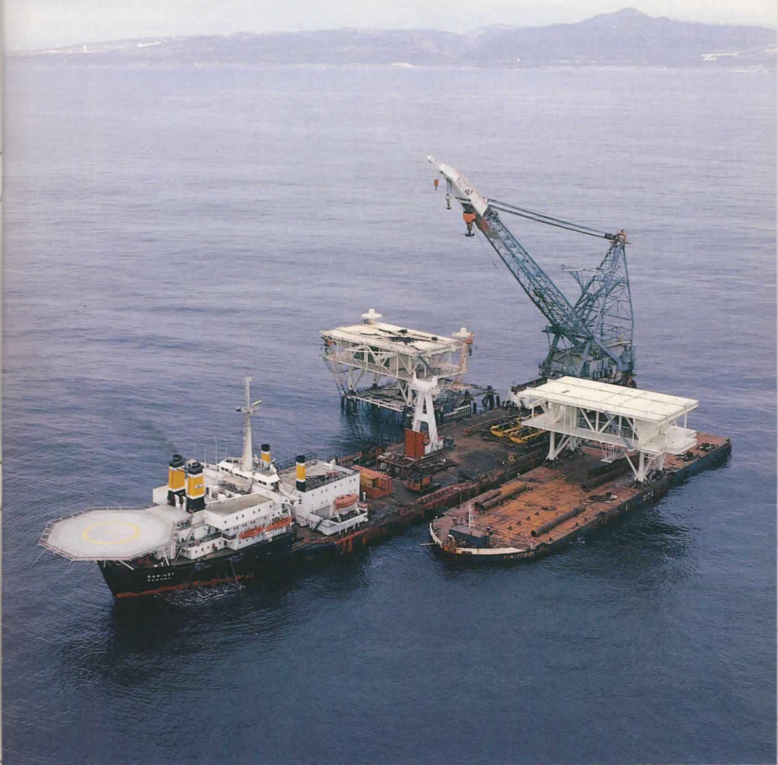
Two decks are installed atop Irene for production and drilling activity. Left, workers prepare to be lifted in "baskets" to the tugboat by crane. Opposite page: Mike Craig (right) talks with Dick Gillen aboard the Sarita before boarding the launch barge to inspect the jacket.
