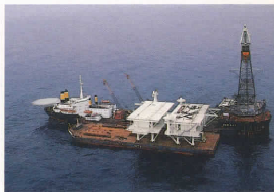
Arrival: Platform Irene’s jacket dwarfs the barge that tows it to its launch point offshore California. At top, the jacket is angled towards the sea in the first stage of the launch. Once secured to the ocean floor, the jacket is ready to receive its decks (above).
