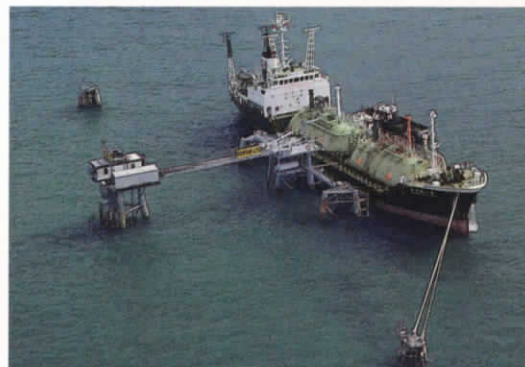
Left, a new wellhead platform just installed by a construction barge in the Yakin North field. Above, a ship takes on liquid propane at a loading facility offshore UOI's Santan terminal.
