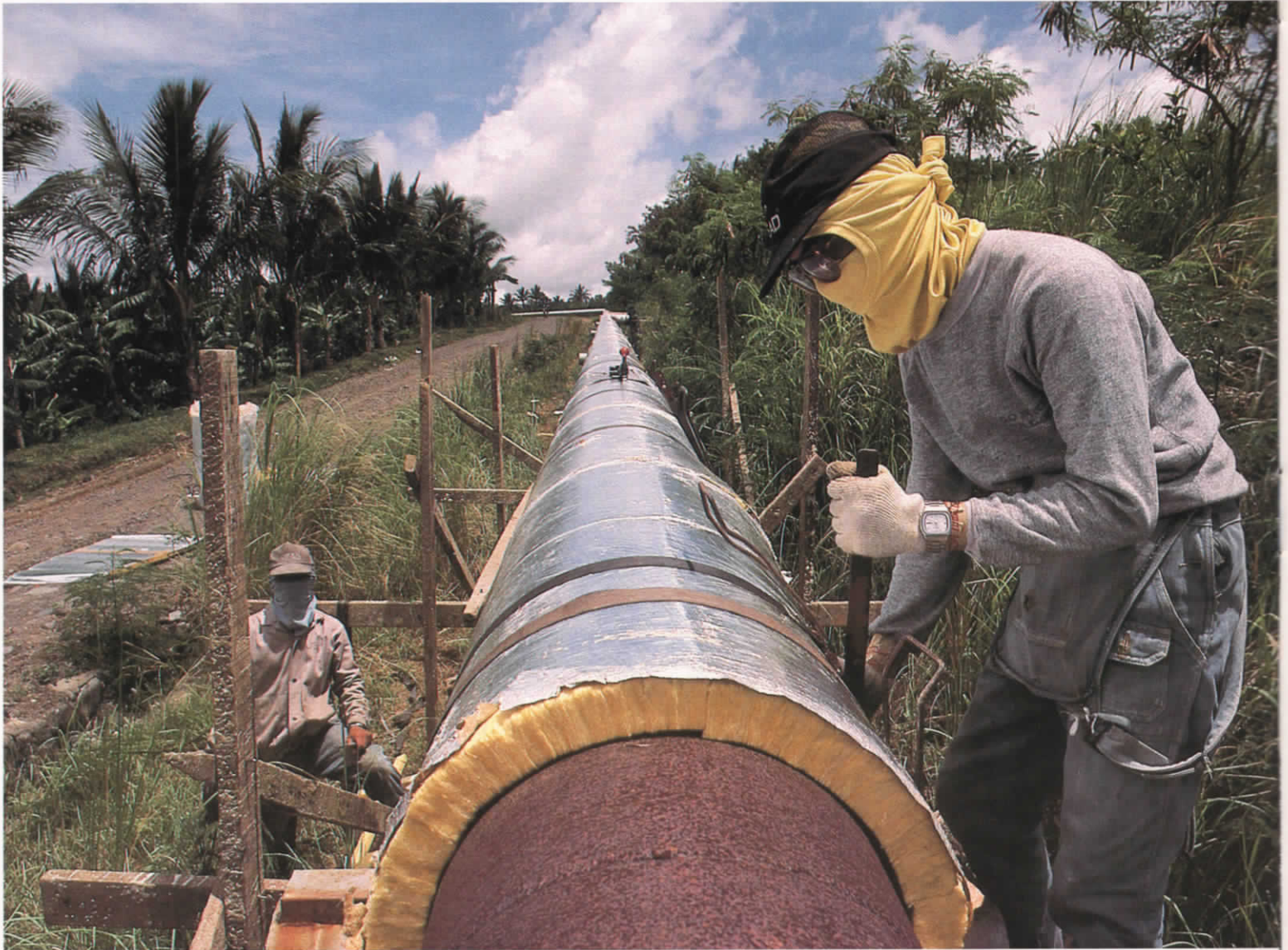
Right, a worker inspects portion of a turbine at one of the Bulalo field's three power plants. Below, workers fit a Tiwi steam pipe with new insulation.
