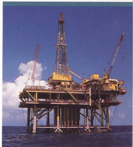
Cerveza set a record for size of platform jackets when it was set in 952 feet of water in 1981. The Chunchulla natural gas processing plant, left and top of page, is operated by UXP, which has interests in 17 such facilities in Texas, Alabama and Louisiana.
