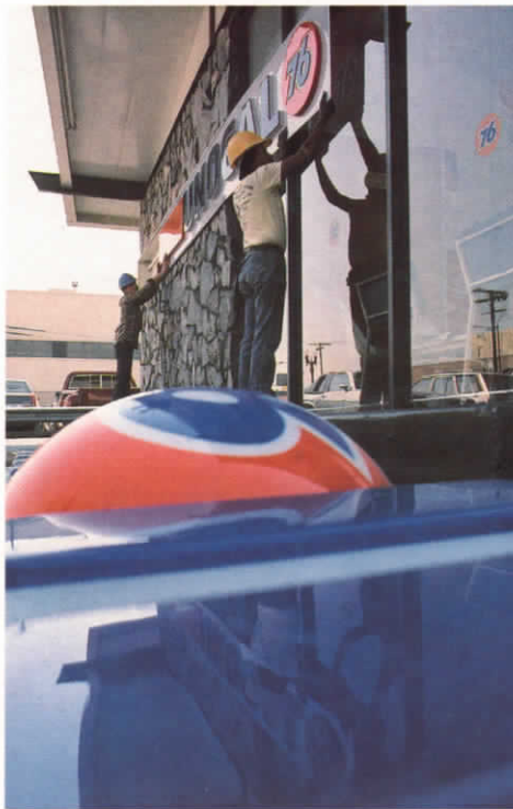
Workers install the new Unocal sign at a Los Angeles service station.
