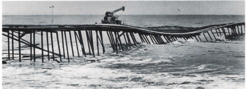
Right, rough seas undermined the old Avila Wharf. (Photo courtesy of the San Luis Obispo Telegram-Tribune.) Twenty months later, the new wharf began operations. Tanker loading and unloading is a round-the-clock operation. The S.S. Coast Range arrived at noon and pulled away with its cargo some 18 hours later.
