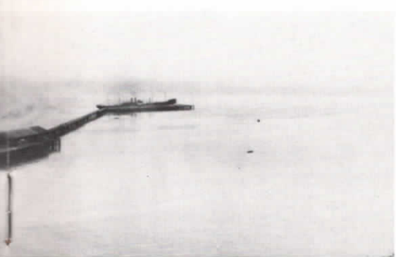
Union's S.S. Coast Range was the first ship to dock at the new concrete and steel Avila Wharf. The old wooden wharf, built in 1914, collapsed in a storm in 1983.
