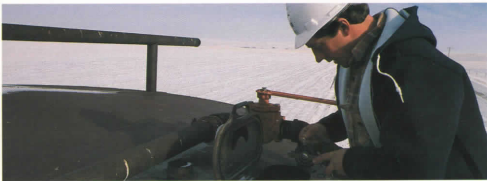
Above: Larson insulates a flow line with straw to prevent it from freezing. Below: Checking a storage tank's oil level with a tape measure.
