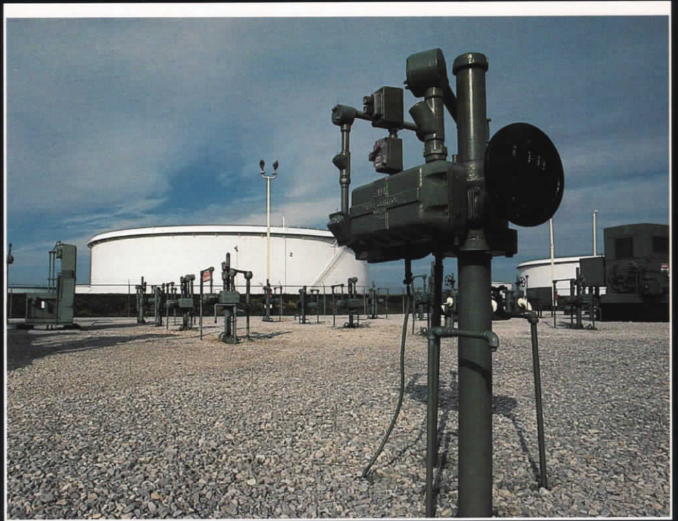
Right, valves and pumps at Chicap's Patoka station move crude oil in and out of pipelines and storage tanks. Below, storage tanks for the Ute pipeline near Moab, Utah. Center, Ron James (left) and Dick Wilkins inspect incoming crude oil lines on the Whitecap pumping platform. Bottom of page, the pump station built at Van, Texas in the early 1930s is still operating.
