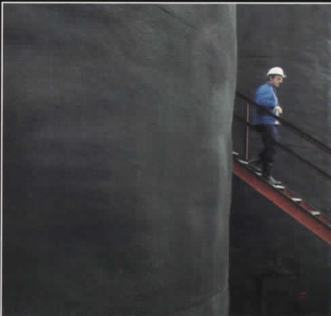
Above: The coal conveyor heads from the crusher toward Obed's processing plant. Right: Bitumen solidifies at less than 70 degrees F., so all piping and storage tanks at the heavy oil project must be heavily insulated. Far right: Workers drill a new test well at McLean.
