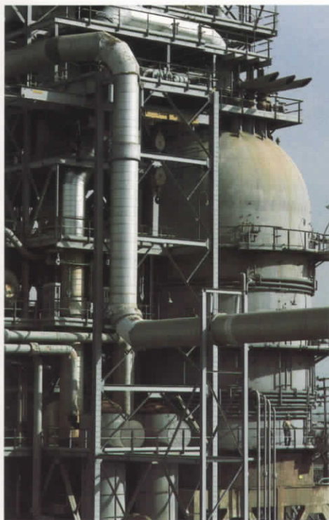
The fluid catalytic cracker (above) uses lanthanide-derived catalysts to squeeze more gasoline out of heavy crude. Every color TV on the market uses lanthanides in its picture tube (right).
