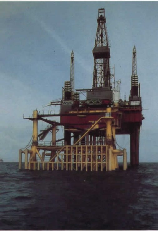
The Hoorn platform jacket awaits construction of the decks and process equipment, while development wells are drilled from the jack-up rig in the background. The Helm platform (opposite) shows the completed drilling deck connected by a bridge to the processing decks and living quarters.
