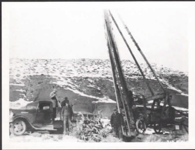
Preparing to abandon a well.
